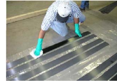
(b) Cleaning CFRP laminates
