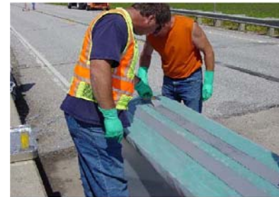
(c) Epoxy application on laminates
