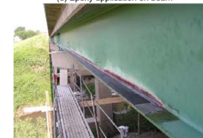
(f) CFRP laminates installed
