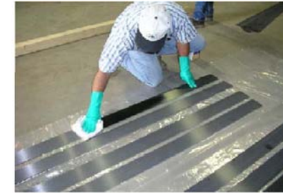
(b) Cleaning CFRP laminates
