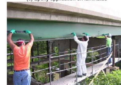
(e) Placement of CFRP laminates (Phares et al. 2003)
