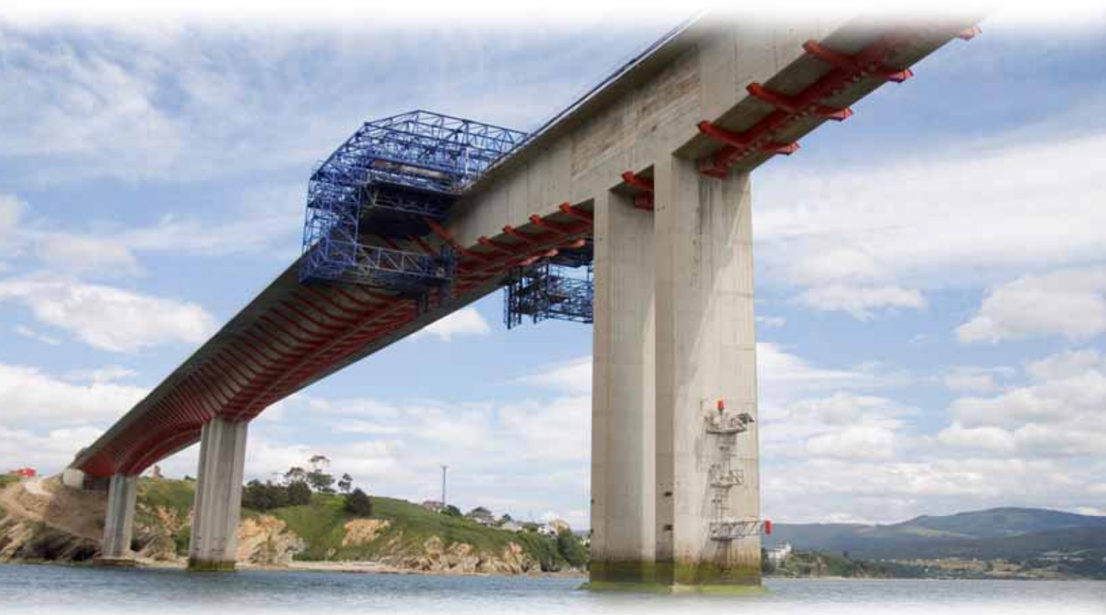
Upgrading of Los Santos Bridge
