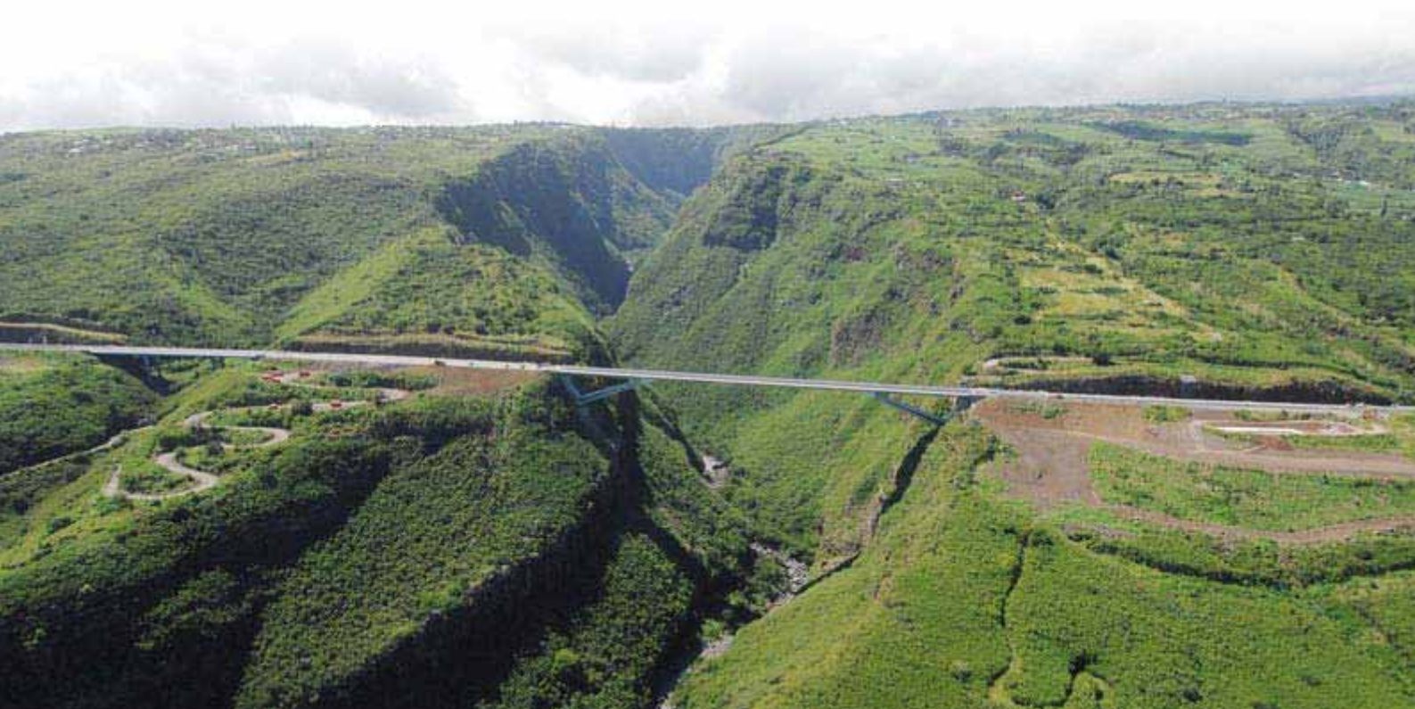
Grande Ravine Viaduct
